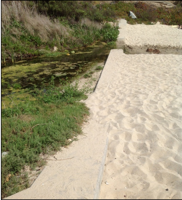
Figure 8. Concrete weir and creek discharge, facing north
