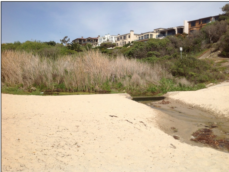
Figure 7. Concrete weir and surrounding vegetation, facing west
